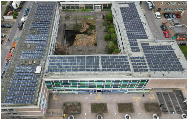
Glyndwr solar array, part of 1800 panel install
